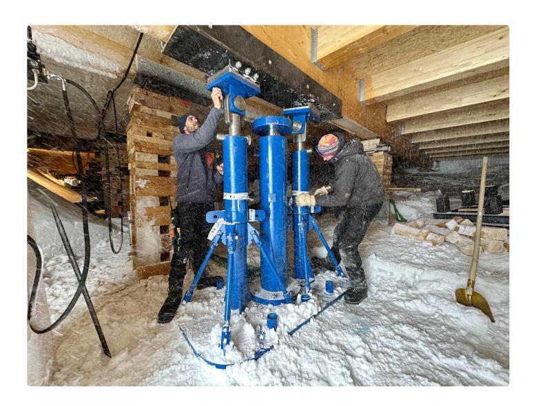
After a full week of getting the station and all its systems back up and running at full capacity, it's time for other major tasks to be initiated. One of the big undertakings each season is leveling the station's annexes. This must be done at the beginning and end of each season to ensure that the building stays level since it rests on a continuous moving surface, the ice sheet.
