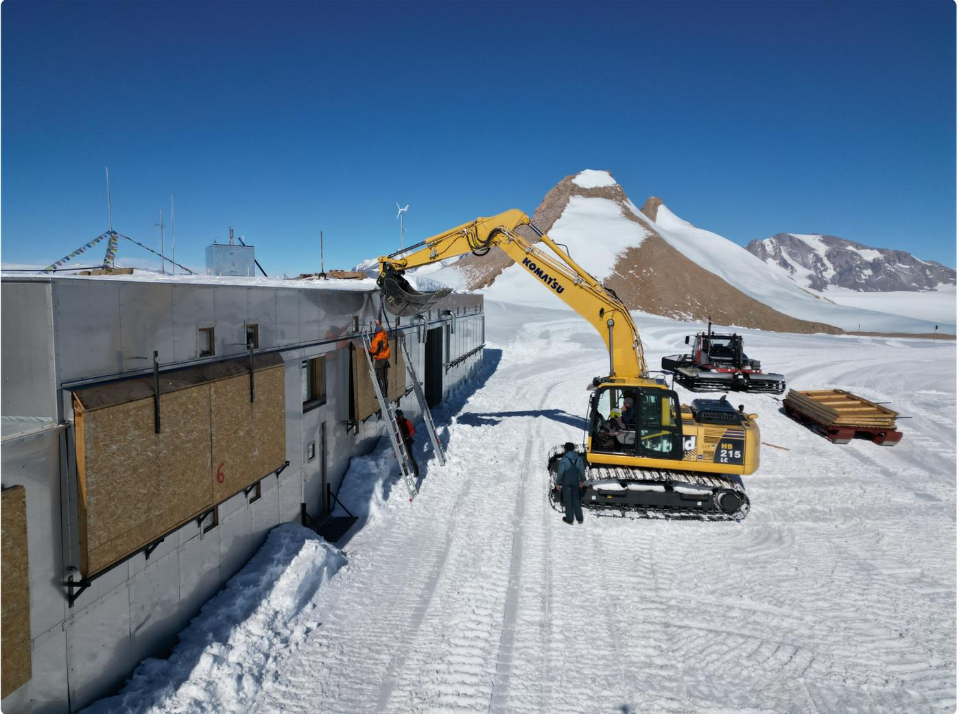
Switching to winter mode involves checking that the electrical and communication systems are working properly, verifying that all scientific instruments are running autonomously so they can continue to collect data, raising the station's annexes to compensate for the movement of the glacier underneath it, covering the station's solar panels, shutting down the snow melter, and draining the water treatment system.
