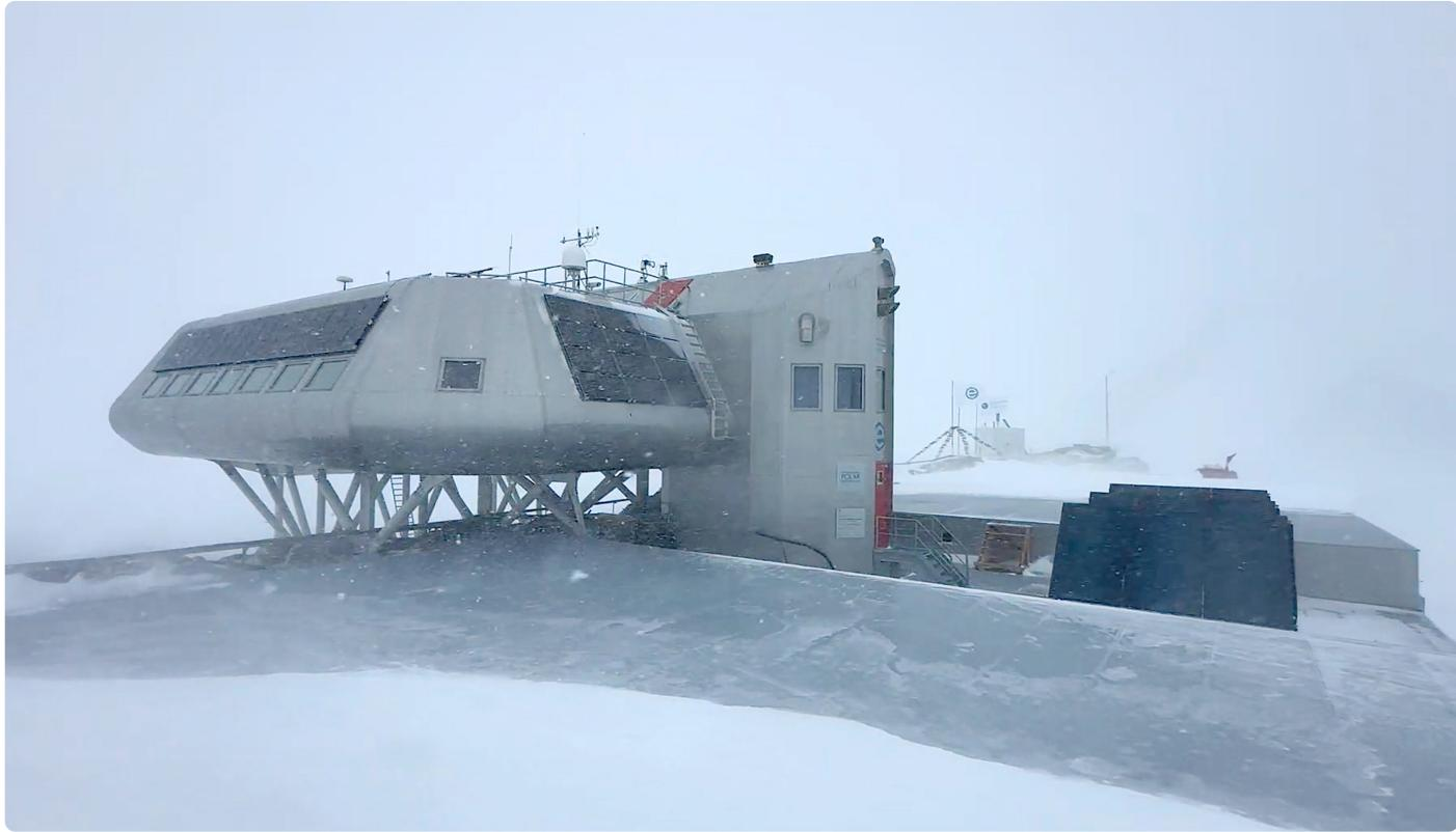
Switching to winter mode involves checking that the electrical and communication systems are working properly, verifying that all scientific instruments are running autonomously so they can continue to collect data, raising the station's annexes to compensate for the movement of the glacier underneath it, covering the station's solar panels, shutting down the snow melter, and draining the water treatment system.
